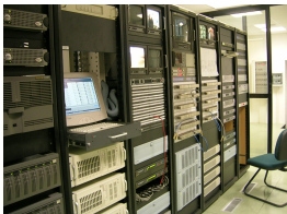
Machine Room Etere
