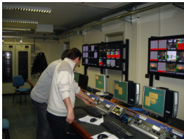
Dove TV Master Control Room
