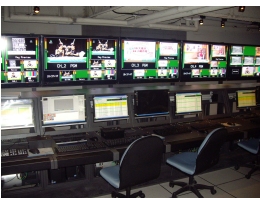
U-Life master control room
