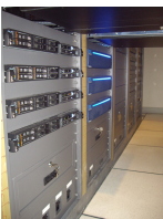
U-Life master control room
