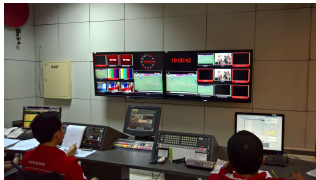
tvOne Etere Installation
